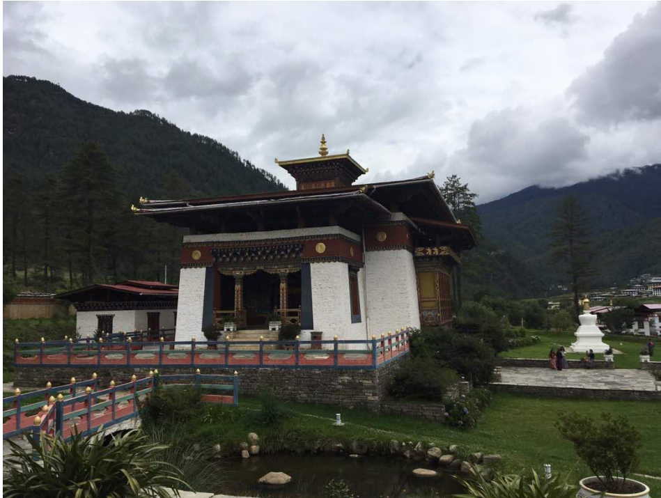
Restoration of the Tara Lhaden Zhingkhram Lhakhang at Pangrizampa, Thimphu
