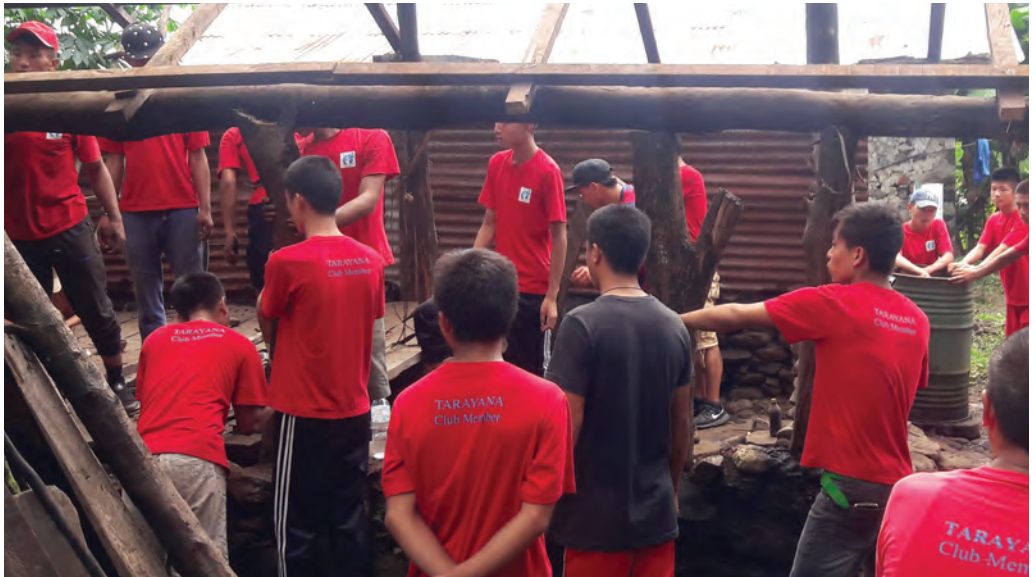
Tarayana Club members of Samtse College of Education actively volunteering to construct a house
