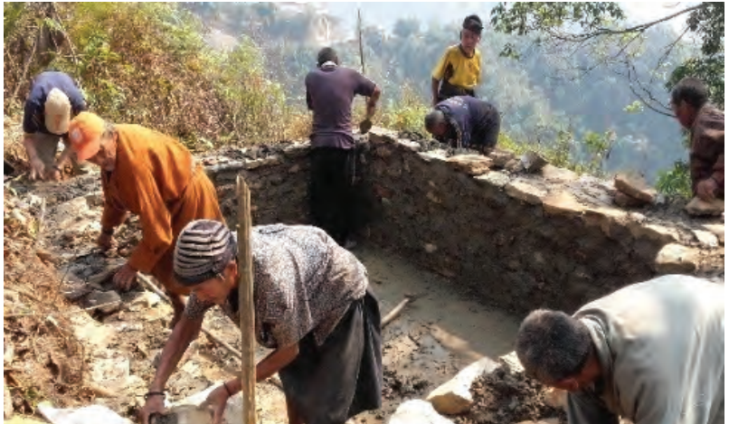
Water tank construction at Migkuri village, Pema Gatshel
